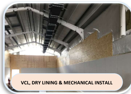
INSTALLATION OF INSULATED ROOF CLADDING
